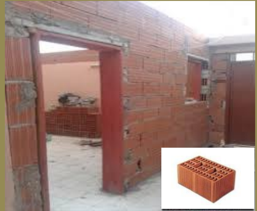
Thermolight block (U-Value 0.08-1)
